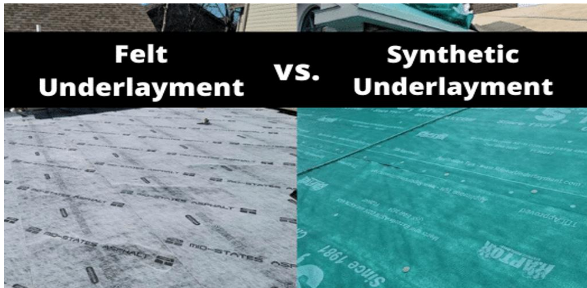
Figure 1: Asphalt-Saturated Felt and Synthetic Underlayment Fabrics (Source: properroofing, 2021)
