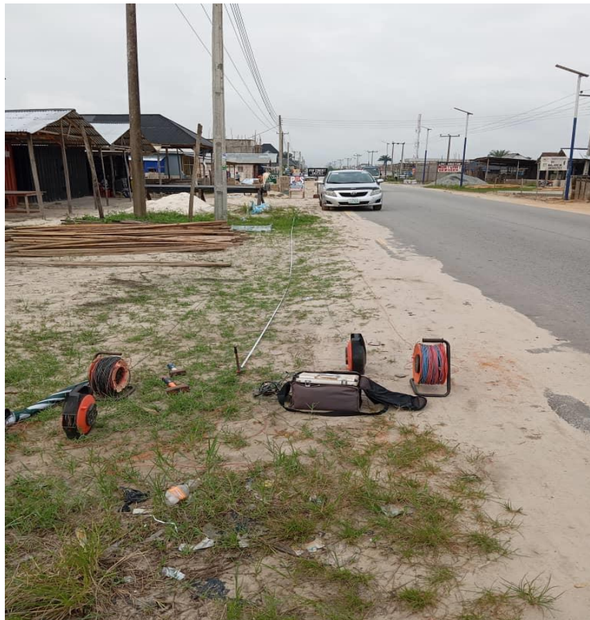
Plate 2: Equipment setups along Ofuoma express way
