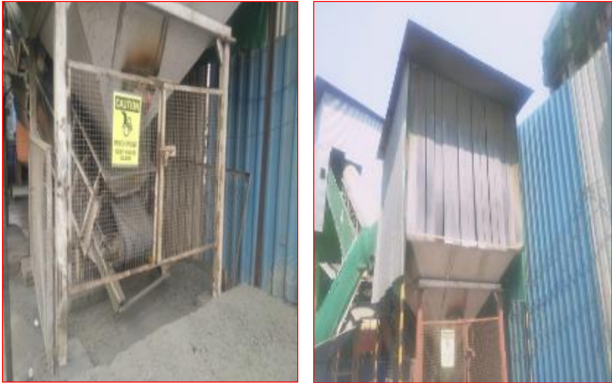
Fig 1 Safety precaution of plant
